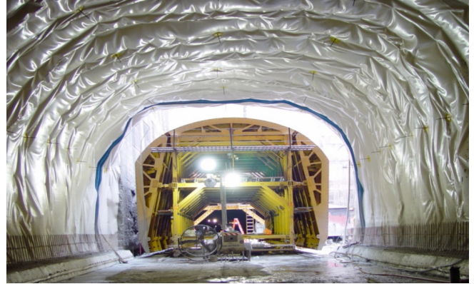
Figure 1. Waterproofing installed, final lining installation ongoing.
