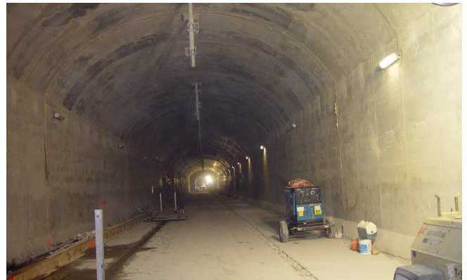
Figure 2. Final tunnel lining in place and finishing out.
