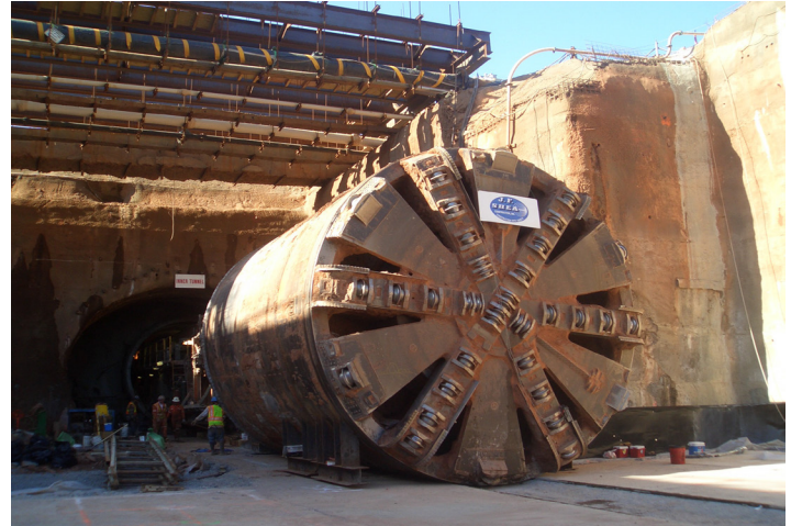
Figure 1. TBM walk-through at the 3E Station cut-and-cover box.
