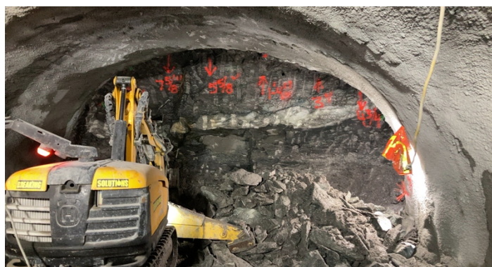
Figure 1. Top Heading Excavation of the New Passageway Tunnel.
