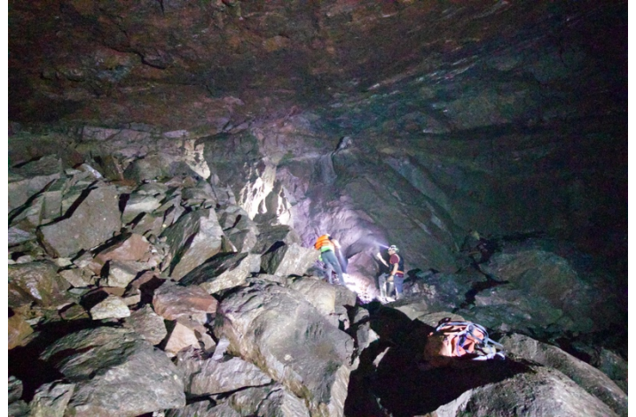
Figure 1. Resulting Cavern from tunnel collapse.
