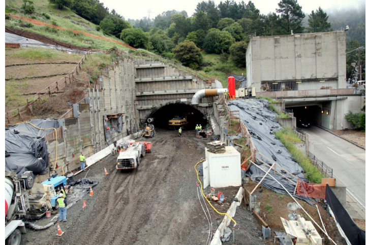
Figure 1. Existing West Portal of the 3 rd bore and new 4 th bore.
