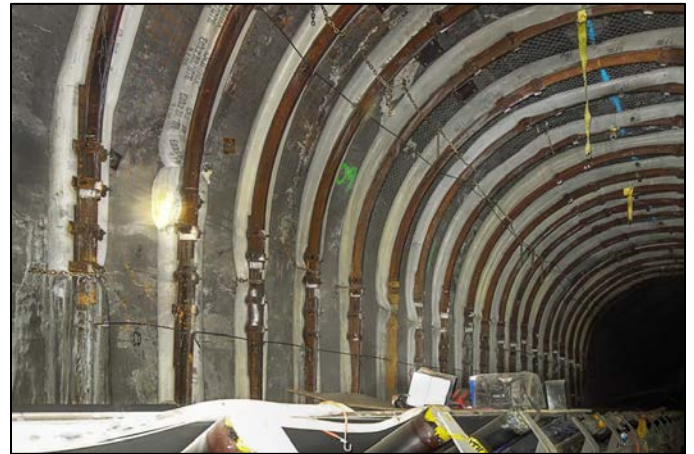
Figure 13. Completed tunnel section with TH steel sets.
