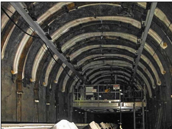
Figure 12. Elevated work deck over the running conveyor belt.
