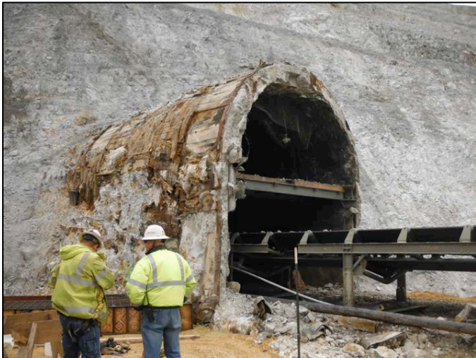
Figure 2. C6 Tunnel, partially unearthed during open pit mining activity
