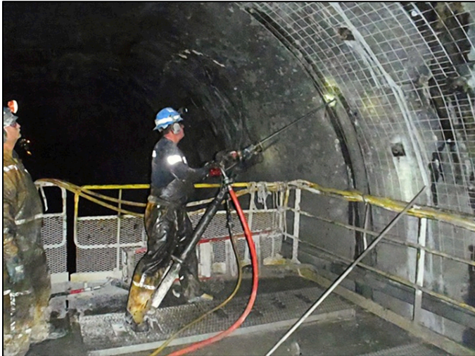
Figure 11. Bolting work deck.
