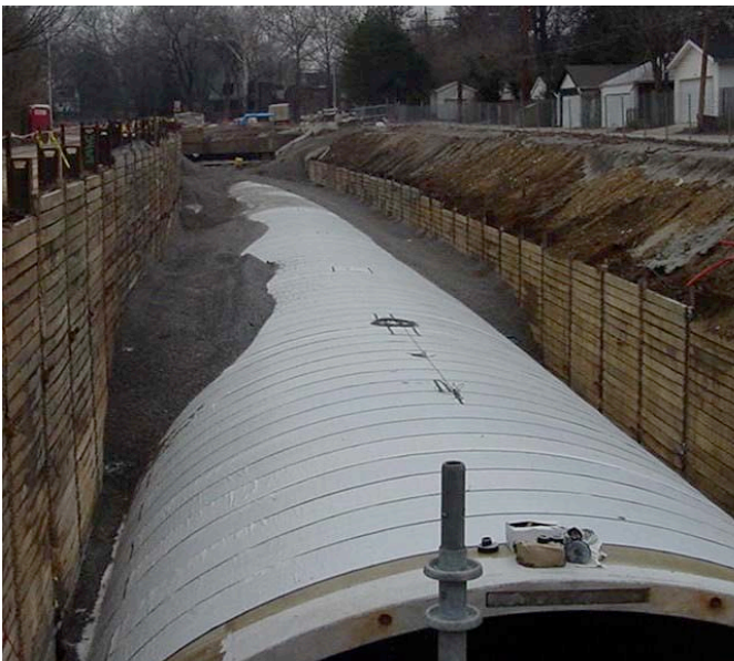
Figure 1: Waterproofing membrane installation on precast tunnel tops
