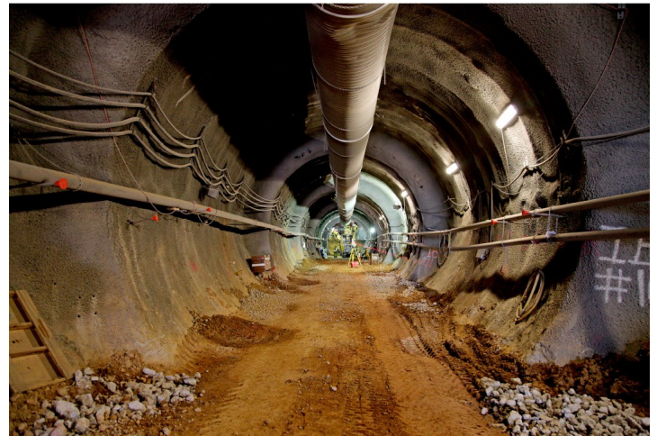
Figure 1. NATM tunnel excavation, April 2010.
